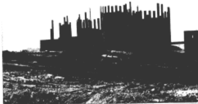
Figure 5: Installation of Circular Cell Cofferdam
