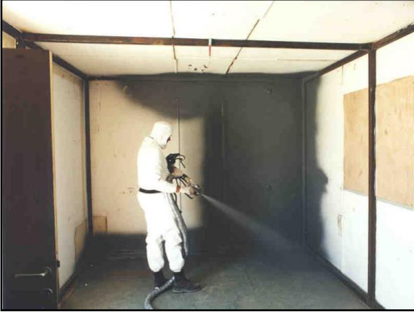
Figure 3: Pre-test elastomer application, TAFB, 2002
