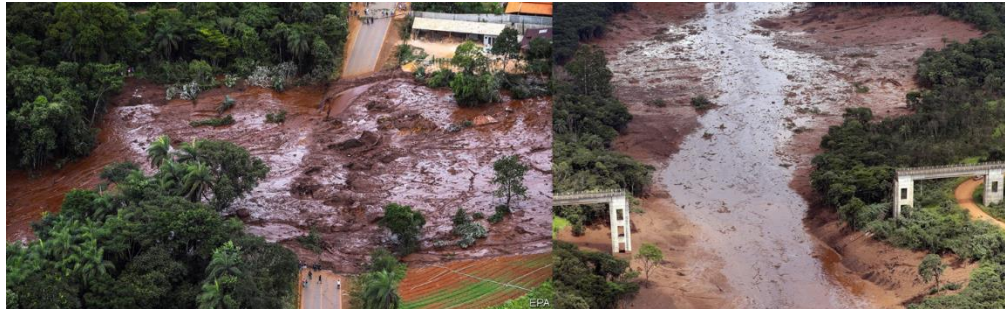
Fig. 10. An aerial view shows a destroyed bridge 2019 after the dam burst, Brazil.
