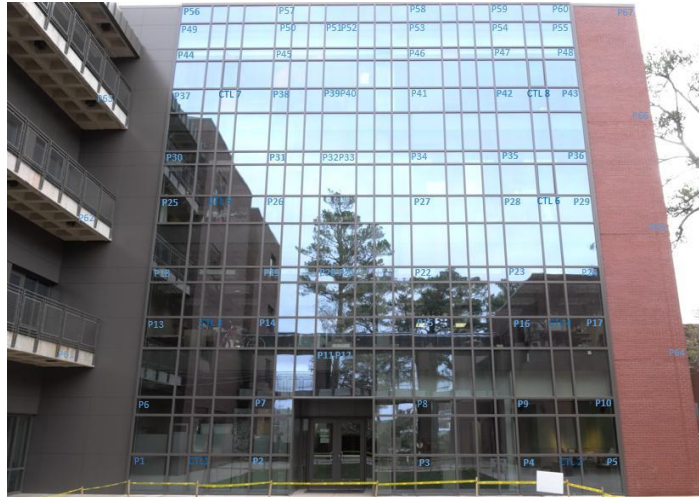
Figure-2: Building Façade and Point Map
