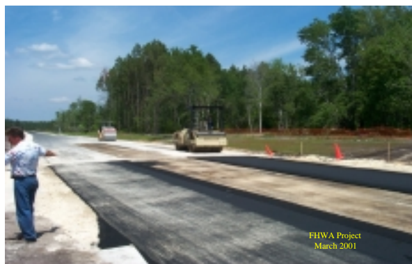
Figure 1: Case Study Project
