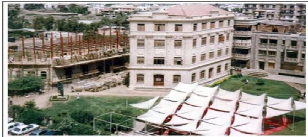
Figure 4: Completed East wing in 2001 with work progress on West wing
