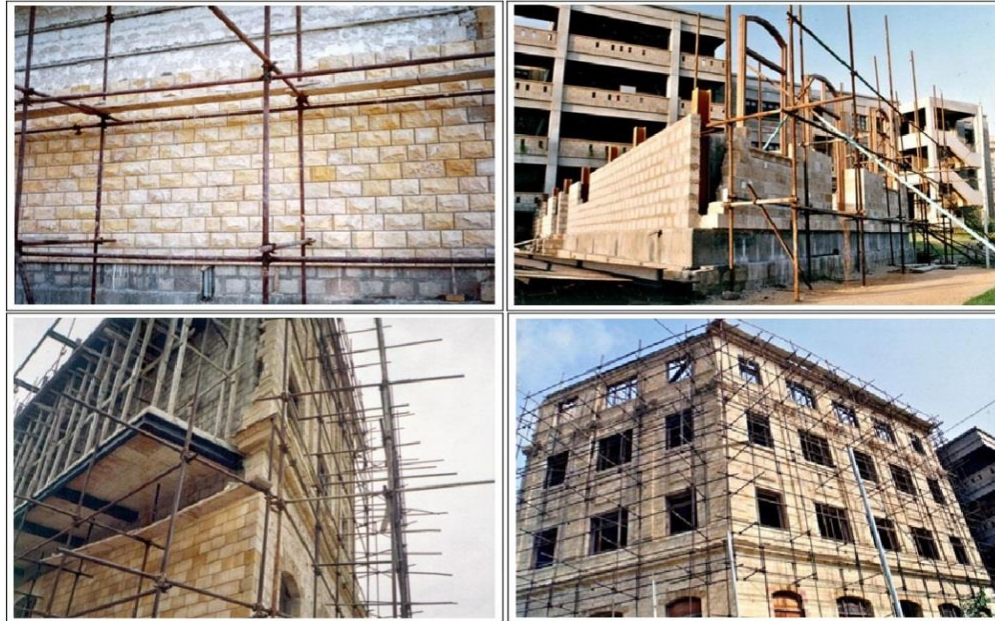
Figure 2: Stone facing, inner and outer walls for masonry of East wing
