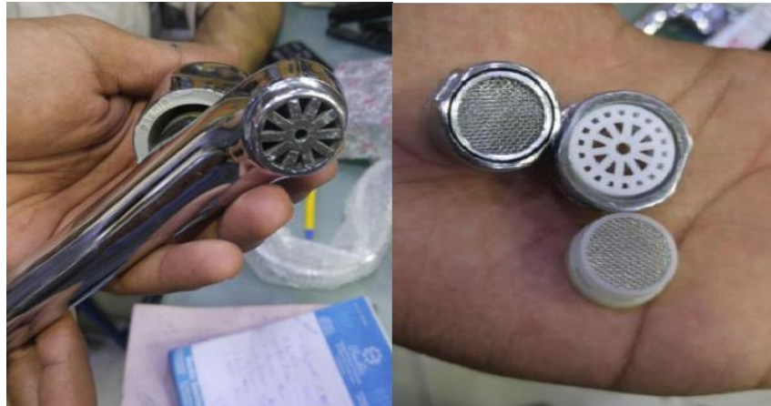
Fig 6. Three Types of Aerators
