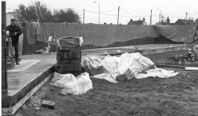
Figure 1: Single-storey, UK built, esh unit as of November 2001
