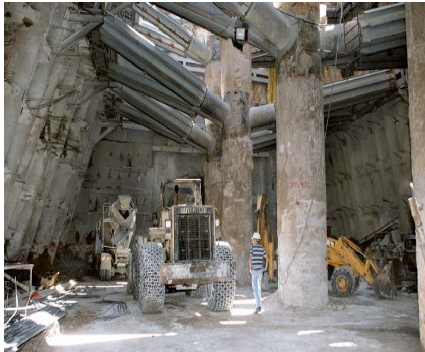
Figure 5: Excavation at Bottom Level
