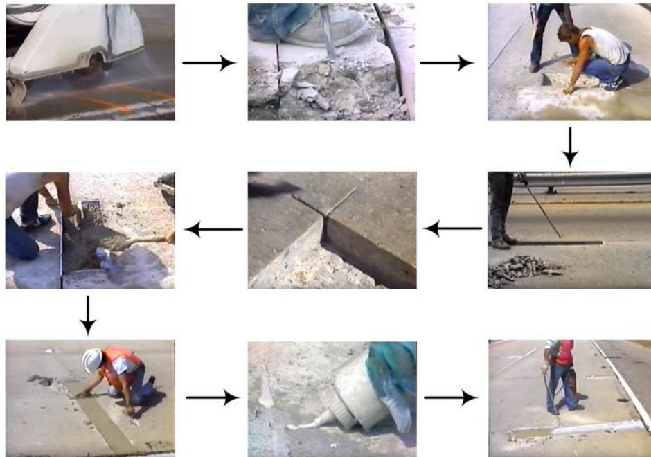
*Figure 1 Mill-and-Patch repair method sequence (Source: FHWA, 1994)*
