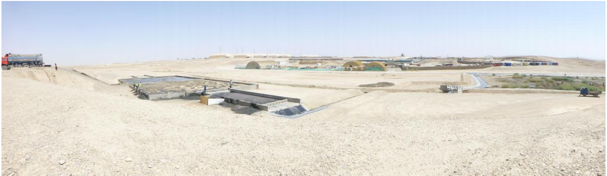
Figure 2. Reed bed sewage facility panoramic (photo by Mr. Alan Newcombe, AECOM)
