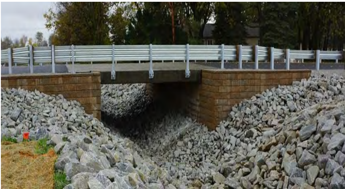
Figure 2: One Span GRS-IBS Bridge (FHWA, 2017)
