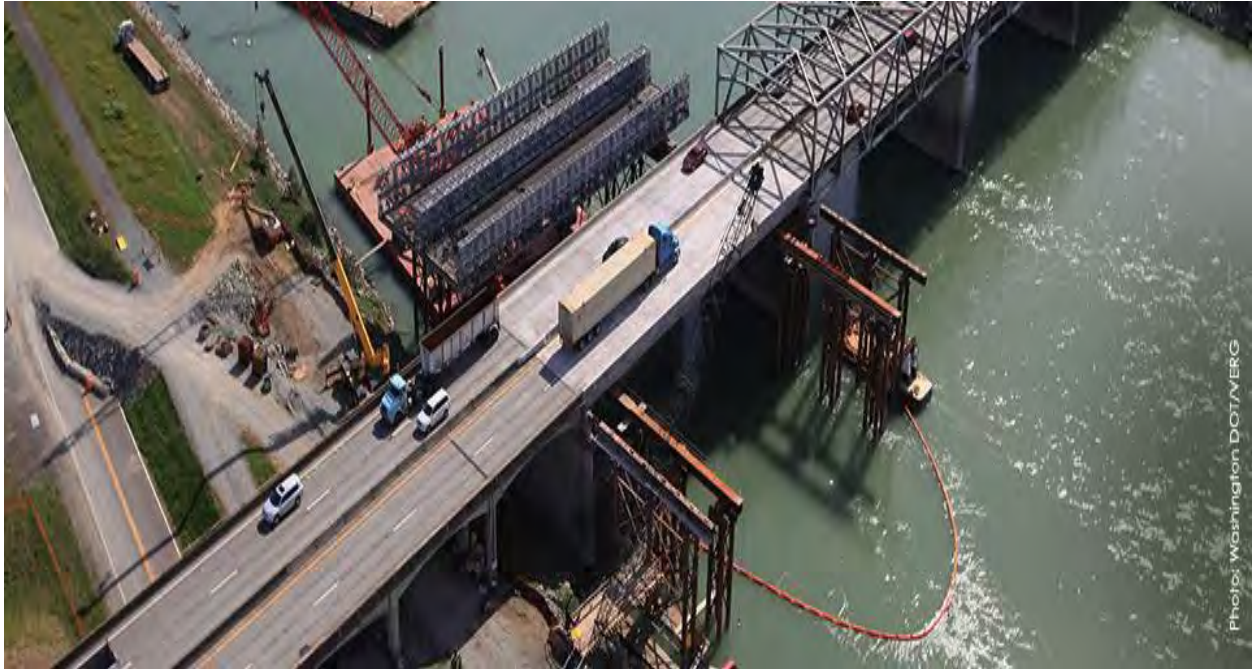
Figure 3: SIBC Construction Project by Washington State DoT (FHWA, 2017)
