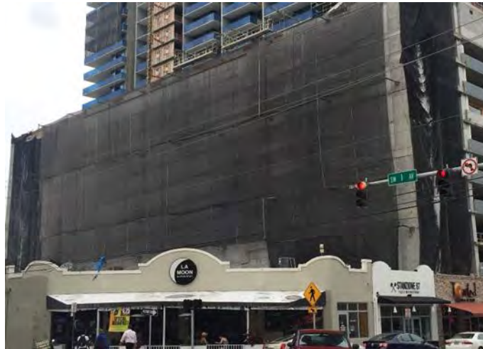
Figure 4: Vertical Netting System
