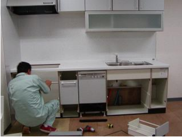
Figure 3: Kitchen unit installation work
