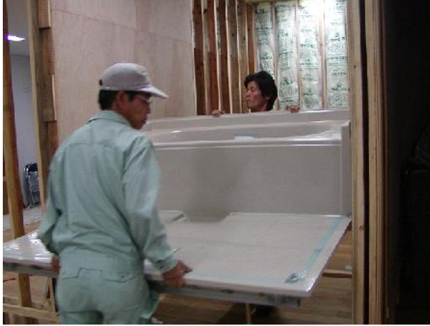
Figure 2: Modular bath unit installation work
