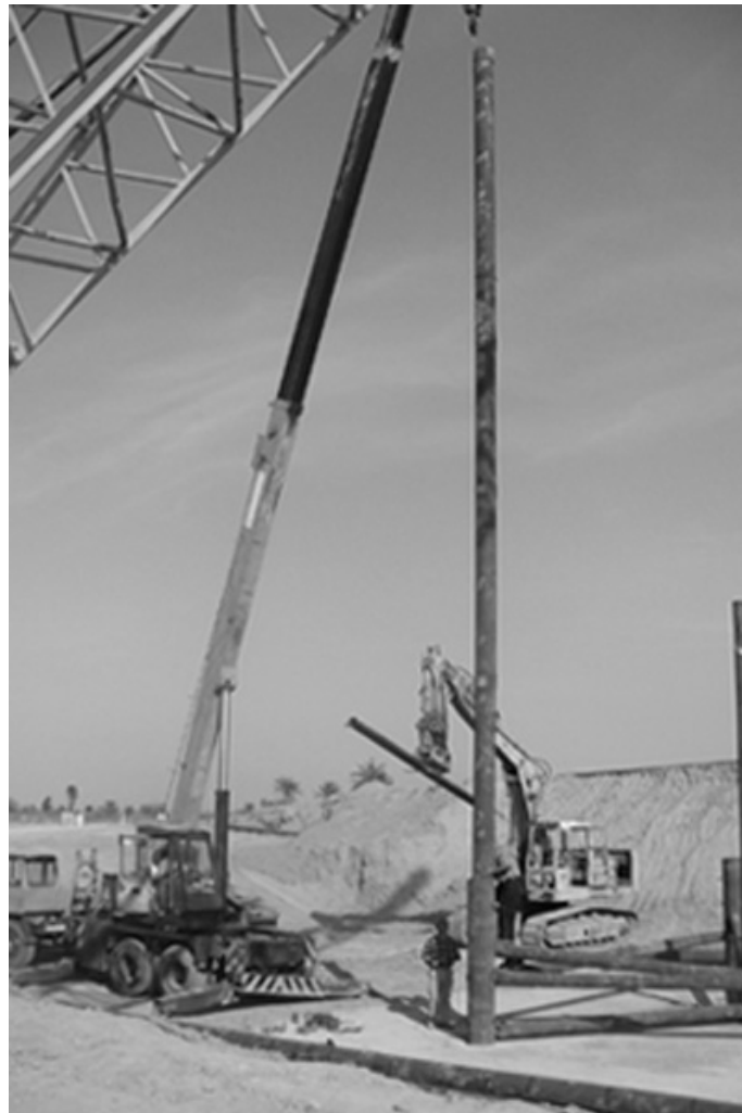
Figure 3: driving pipes through pile template
