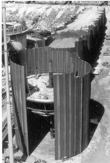
Figure 2: European template and cell dam installation
