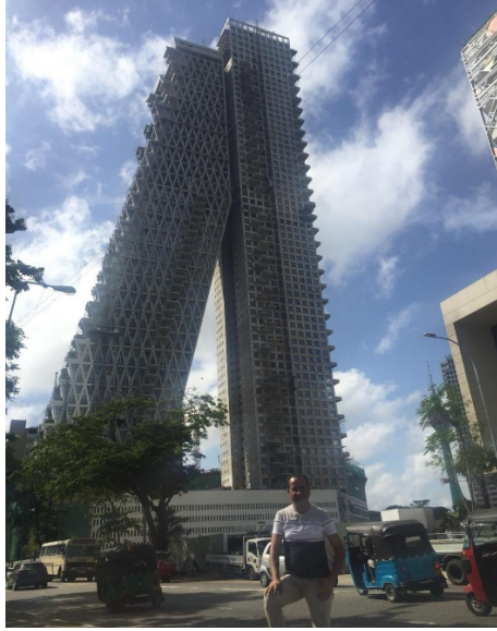
Fig. 1. Upcoming Hyatt Regency in Colombo, San piling, 2016
