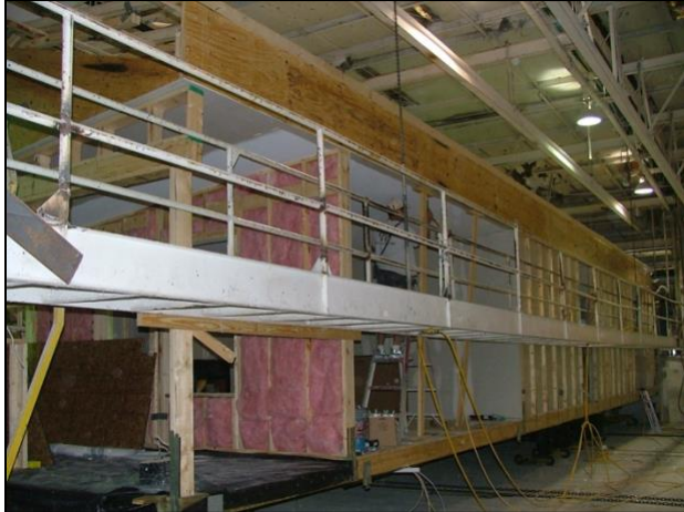
Figure 5: Improved end and marriage wall stud dimensions (2x4 and 2x6) and maximum spacing (Draper, 2005)
