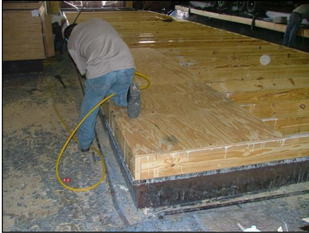
Figure 3: Improved sub-floor sheathing ( \frac{3}{4} " laminated and fastened to 2x10 floor joists (Draper, 2005)
