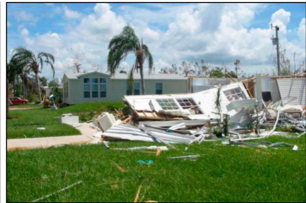
Figure 2: Comparison of hurricane damage to pre-1994 HUD and post-1994 HUD manufactured housing (FMHA, 2004)
