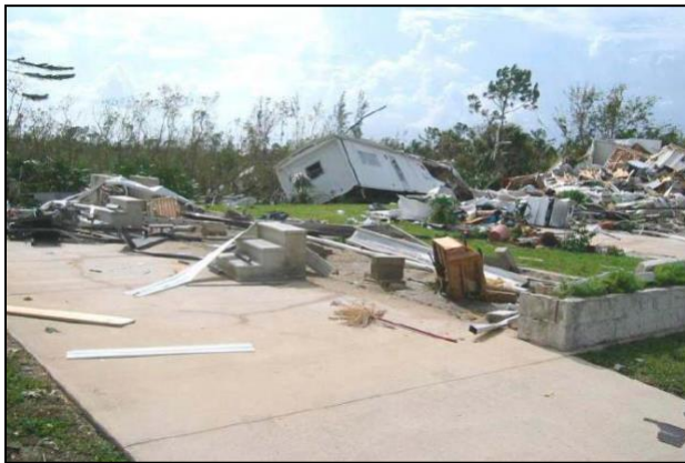
Figure 1: Hurricane damage to pre-1994 HUD manufactured housing (FMHA, 2004)
