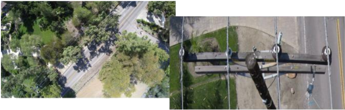
Figure 4: Distribution Line Inspection
