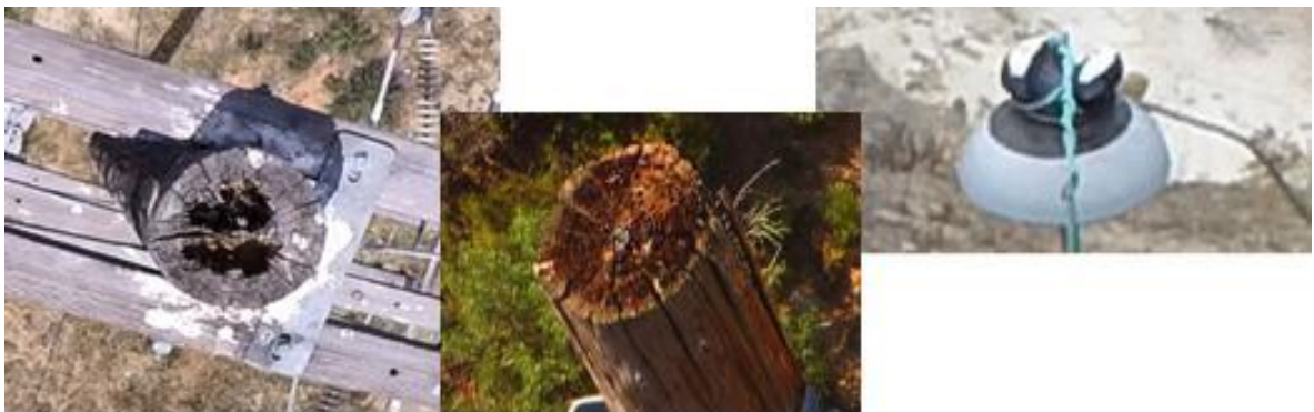
Figure 3: Pole Top Inspections
