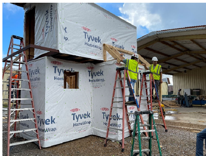
Figure 4. Students install weather barriers on the sheathed walls.
