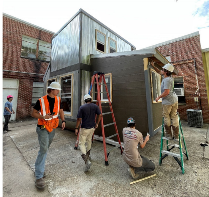
Figure 1. Students completing the exterior finishes at the end of the semester.
