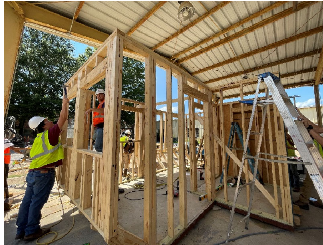
Figure 3. Students engaged in wood framing of the walls.
