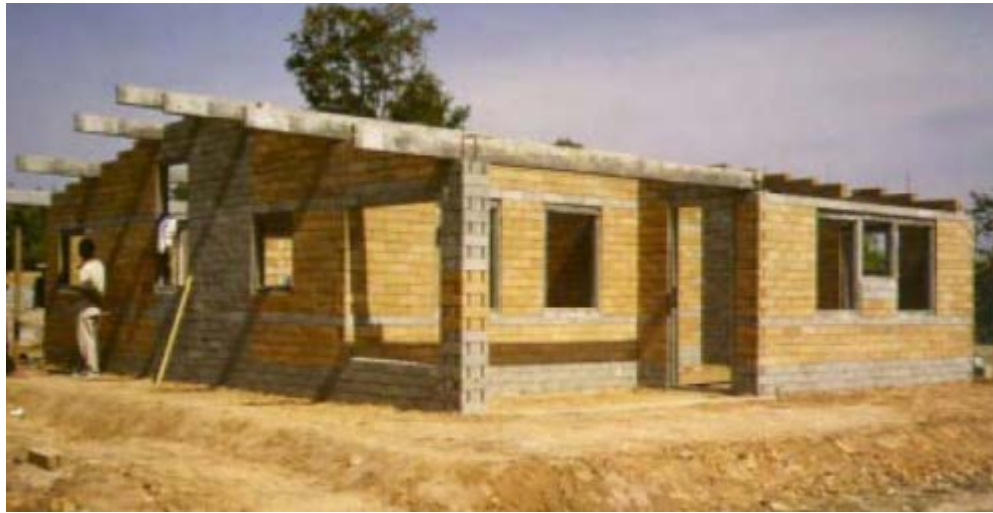
Figure 9 House using interlocking blocks from concrete and laterised concrete
