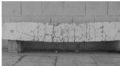
Figure 4: NC Beam after Failure
